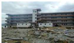
Concrete building survived tsunami, but roof evacuation area inundated by 0.7m water
