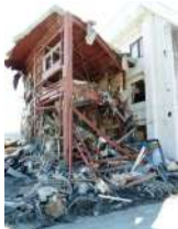
Three-Story Steel MRF collapsed and pushed into concrete building
