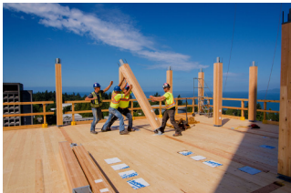
Credit: Seagate Structures
