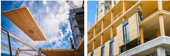
Credit: Seagate Structures
